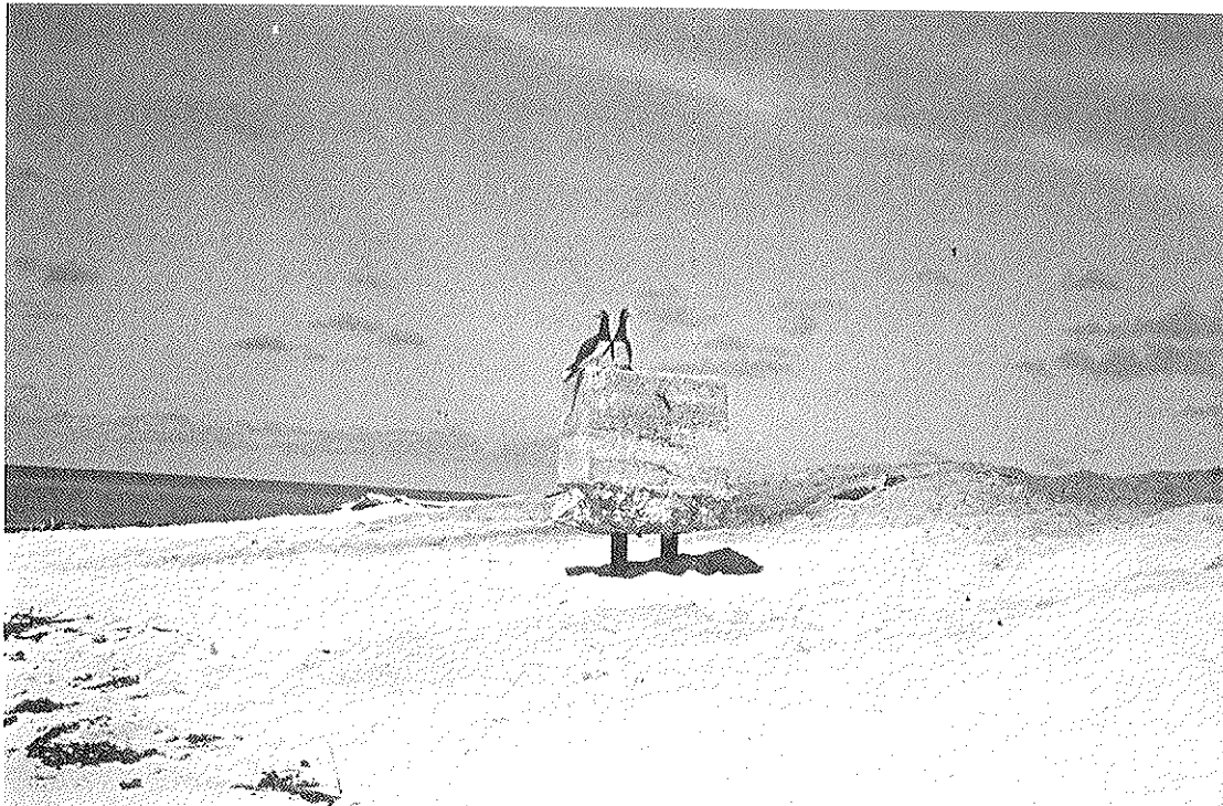
Plate 6. Remains of the 1958 lighthouse.
